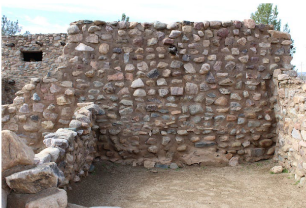
North Building, North side
