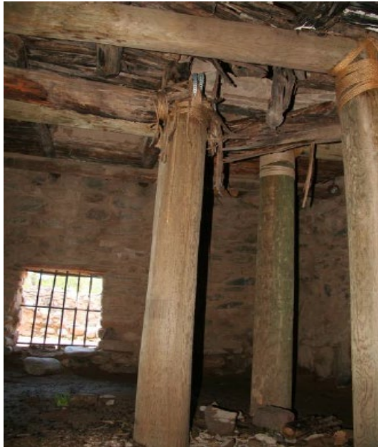
South Building interior posts
