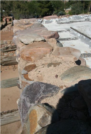
South Building Parapet
