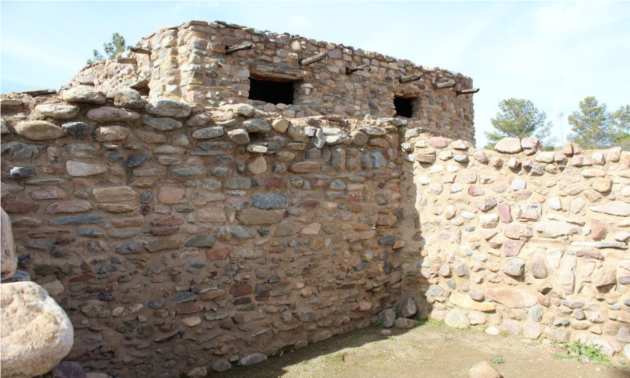
East Building, North Side
