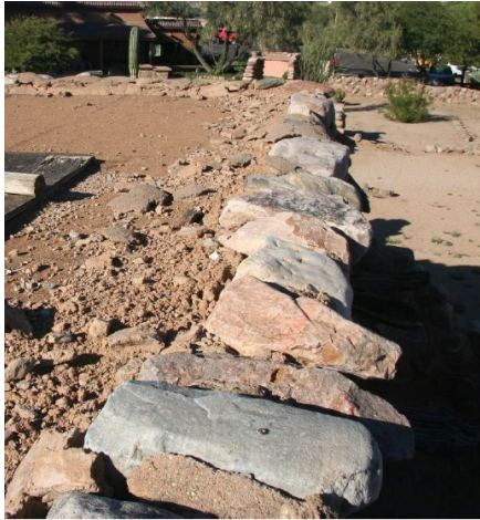
North Building parapet
