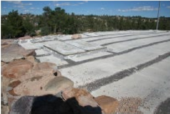
South Building roof
